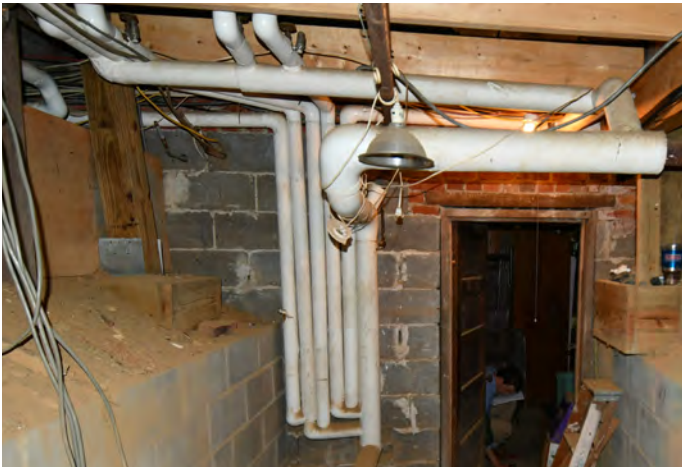
Legacy steam piping to be removed
