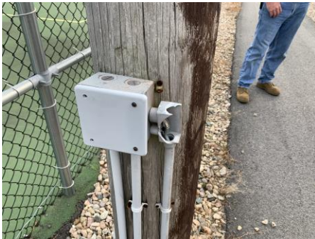
Damaged exposed PVC conduit
