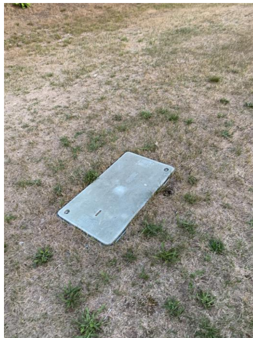
Scoreboard feeder handhole
