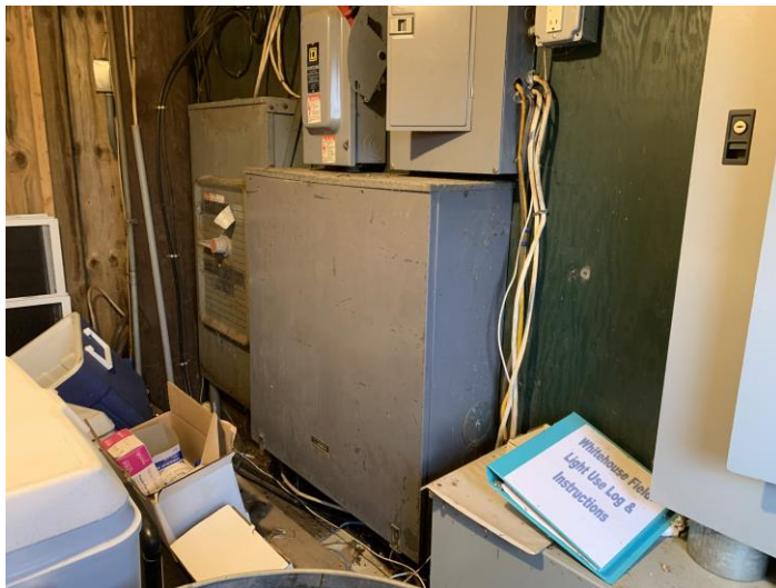
Main electric service panels
