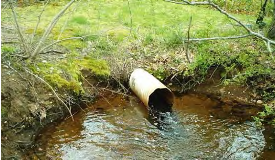
Figure 8 – Culvert Discharging Flow from Minister's Pond to Muddy Creek (18" CMP) with Eel Passage Ramp Substrate (submerged)
