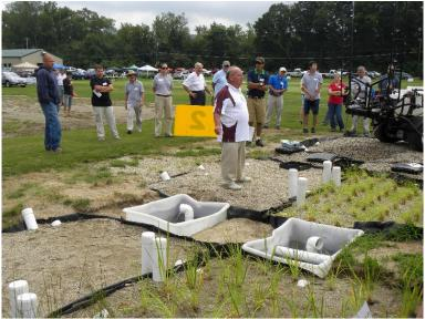
The picture illustrates the area that has been developed at the field plots near campus. These units are being installed for corporations and even as septic systems. They include two chambers that move rinsate water through sand filters and manufactured wetland area where plants help to clean the water. The system is new and is a potential alternative to the wash water recycling units that are now common in our industry.
