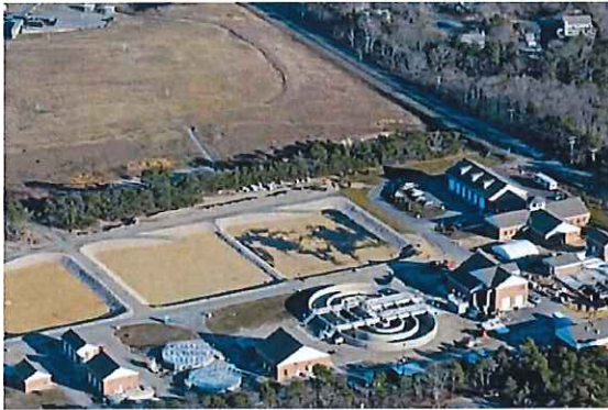
Chatham Wastewater Treatment Plant (1.1 million gallon per day average flow with open infiltration basins)
