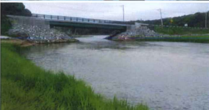
Before (top) and After (bottom) Muddy Creek Inlet Widening.
