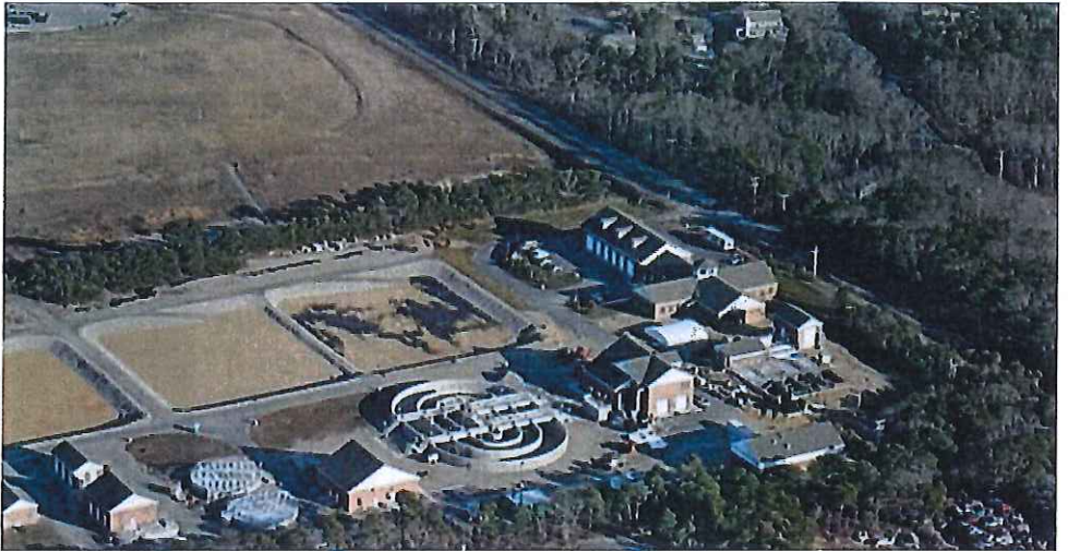
Chatham Wastewater Treatment Plant (1.3 million gallon per day average flow capacity with open infiltration recharge basins)
