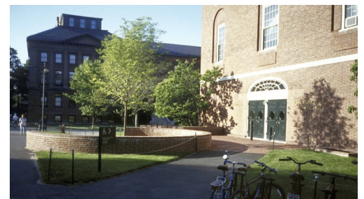
Paine Music Building Expansion, Harvard University: New brick planting wall facilitates the grade transition to allow for universal access at main entry.
