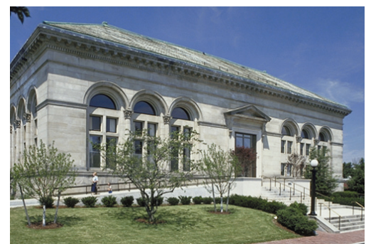
Robbins Library, Arlington MA: New exterior access ramp integrated with historic front entry to library; interior expansion includes strategically located elevator and stairs to accommodate differential floor heights between existing floors and new addition.
