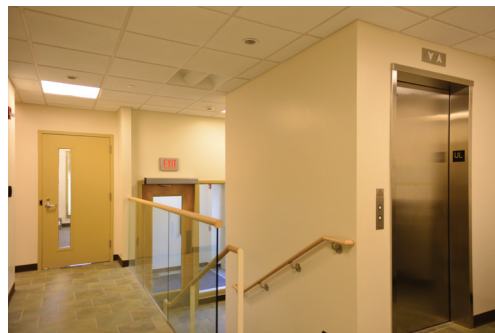
Elevator insertion into Sports Science Dept. Building, FSU
