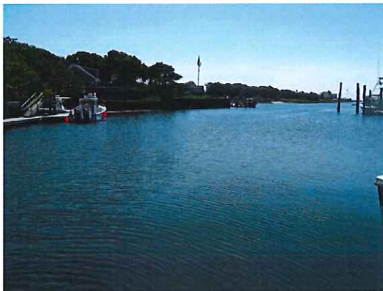
Channel and Private Bulkhead
