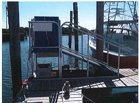
Existing Ferry Access Ramp
