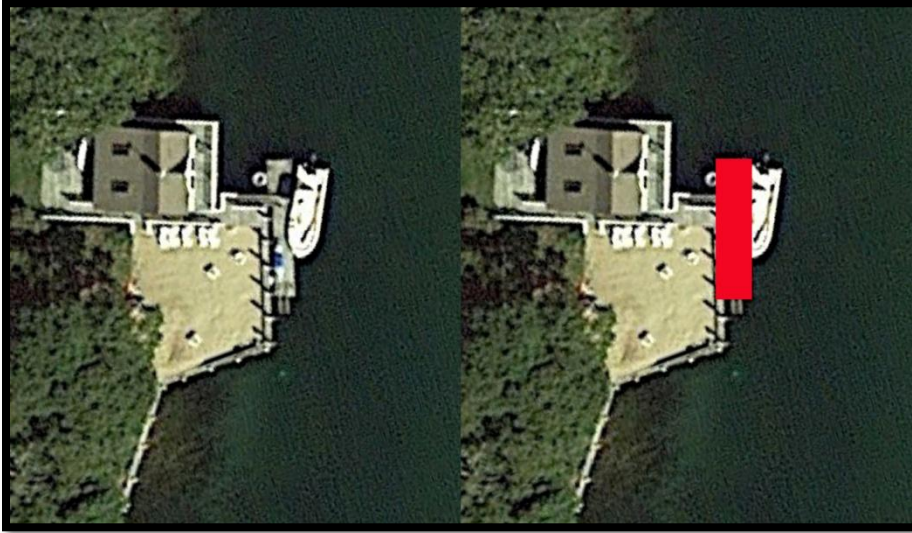
Figure 2. 99 Riverside Dr. Left image is of existing structures, permitted under MA DEP Chapter 91; red box in right image showing proposed floating downweller location.
