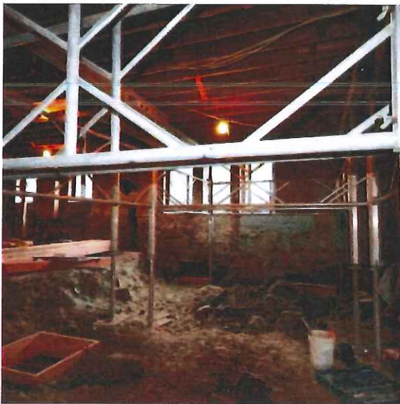
Basement excavation at Bagg Hall in Princeton, MA.
