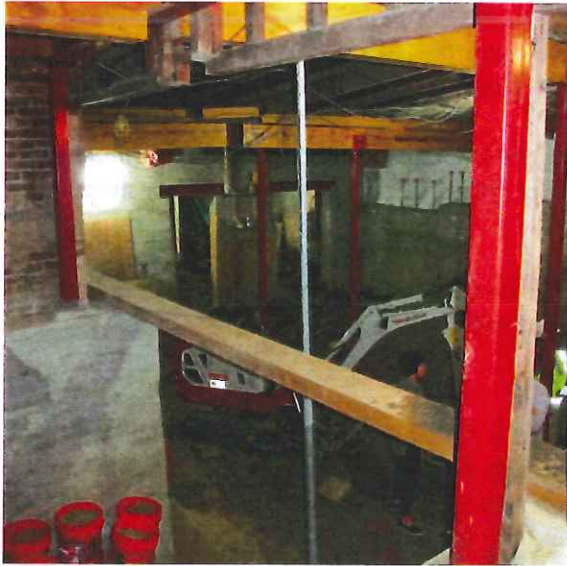
Basement excavation at the Vilna Shul in Boston, MA.
