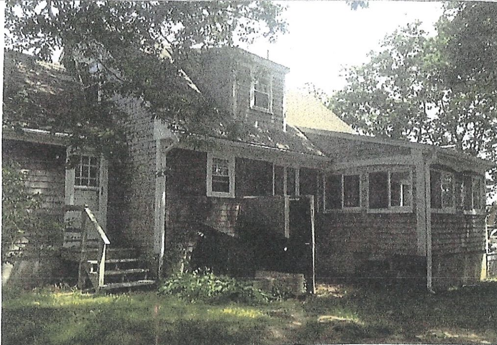
Photo Two Caption REAR VIEW
