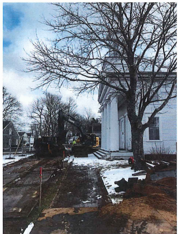
Figure 2 North entry has steps making it inaccessible
