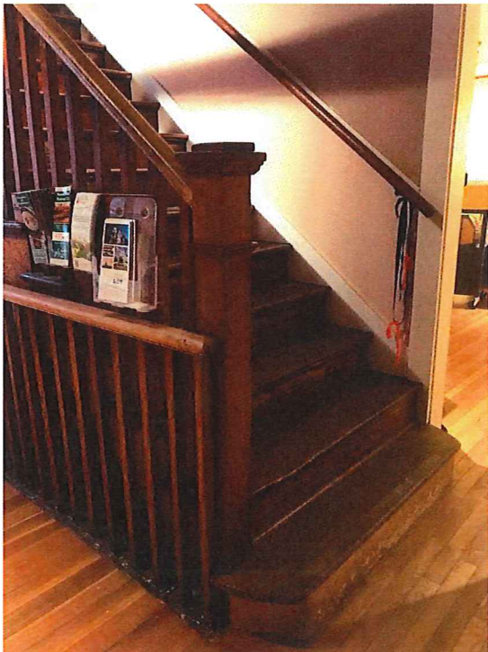
Figure 7 baluster, railing, and newels at stairs are non-conforming
