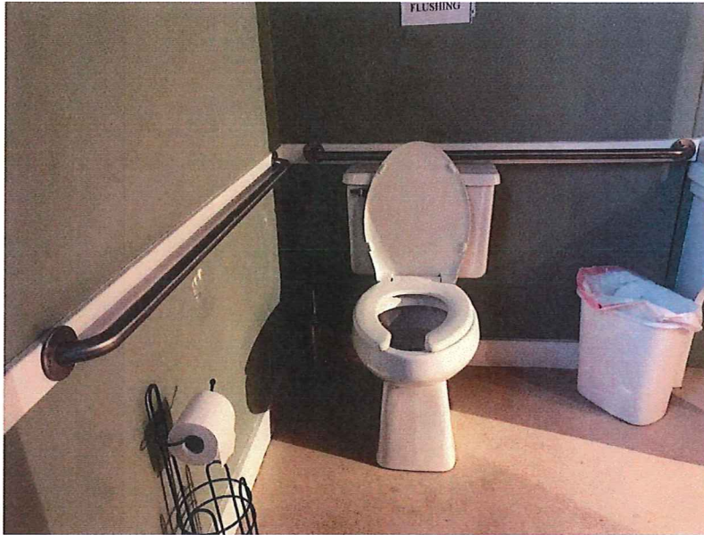
Figure 4 while the toilet room has accessible features, there required clearances for fixtures is inadequate
