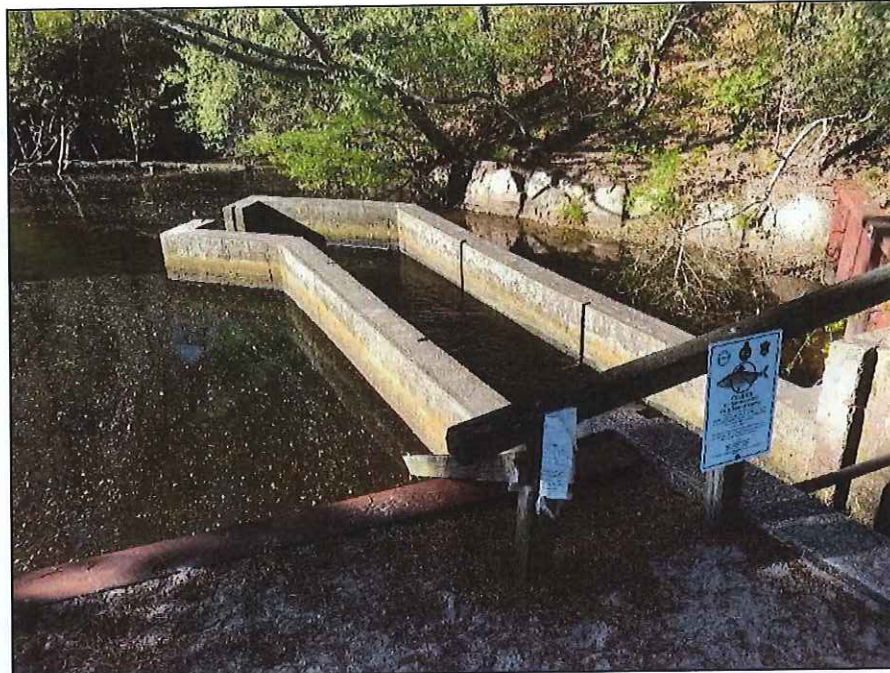
Photo No. 23.: Downstream end / entrance of the fish ladder.
