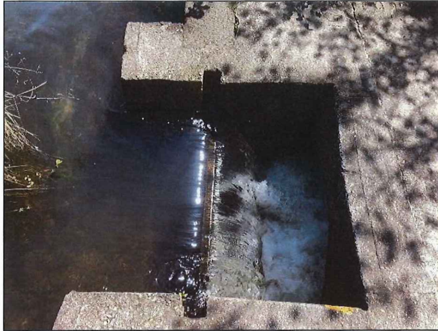
Photo No. 15.: Concrete headwall intake structure.
