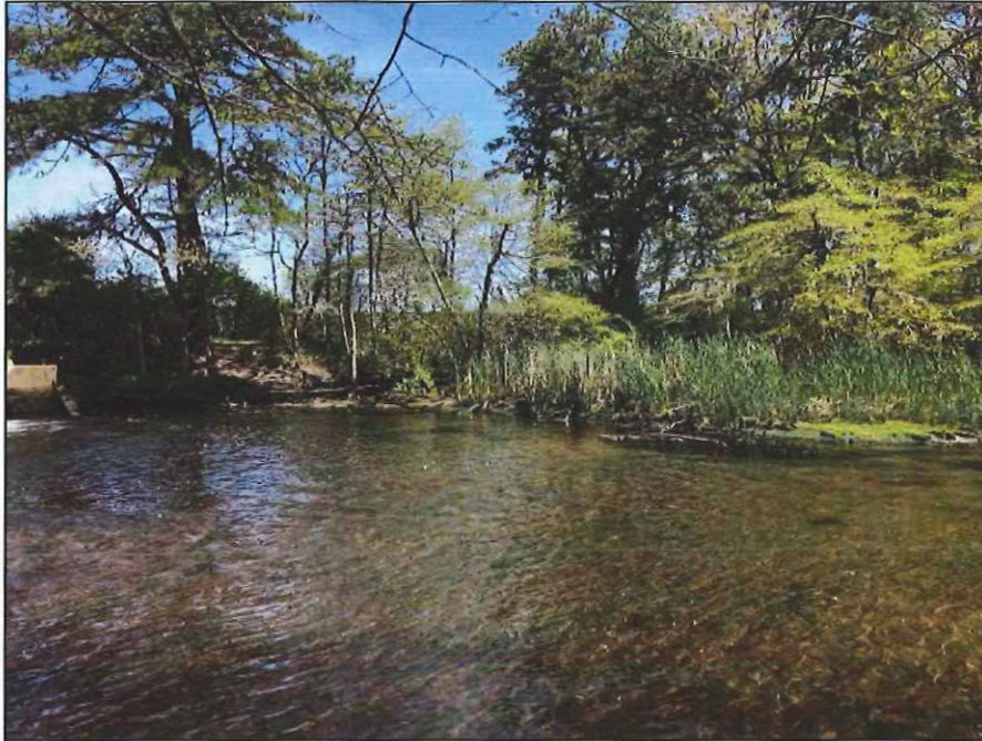
Photo No. 13.: The downstream slope to the left of the spillway discharge viewed from downstream area.
