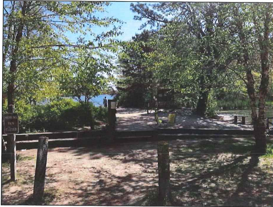
Photo No. 1.: Overview of the Dam from near the right abutment looking left.
