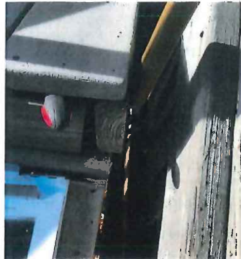
WOOD TO WOOD IS SEPARATING; WOOD TO COMPOSITE IS SEPARATING. HARDWARE EXPOSED.
