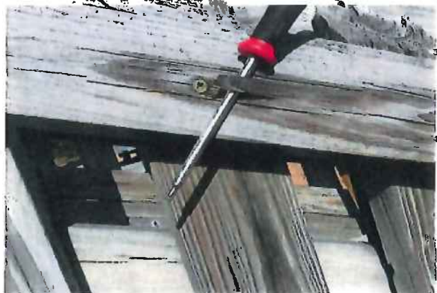
WOOD TO WOOD IS SEPARATING; WOOD TO COMPOSITE IS SEPARATING. HARDWARE EXPOSED.
