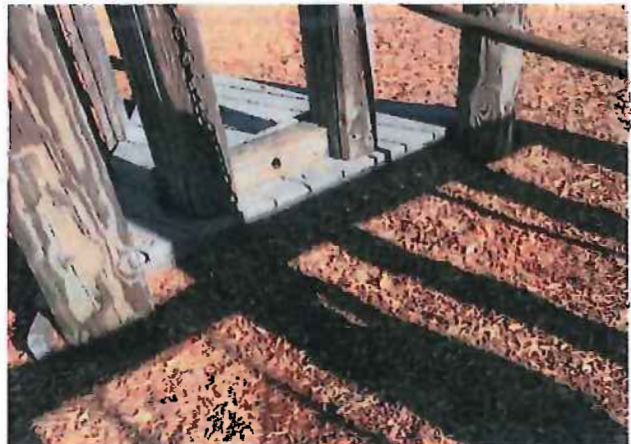
SEE LOOSE HANGING CHAIN – NOT ATTACHED TO ANYTHING.
