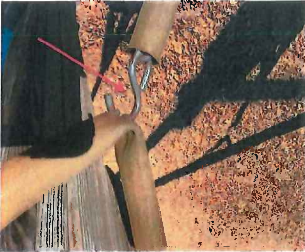
OPEN 'S' HOOK IS WORN AND HAS LOST INTEGRITY.
