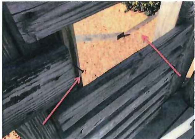
HEAD ENTRAPMENT AND PROTRUDING HARDWARE.
