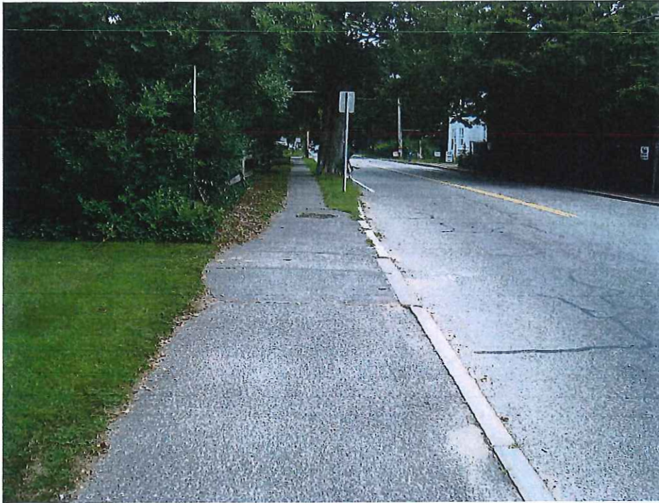
Main Street across from Library
