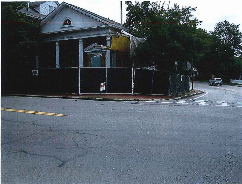
Library on Main Street (During restoration)
