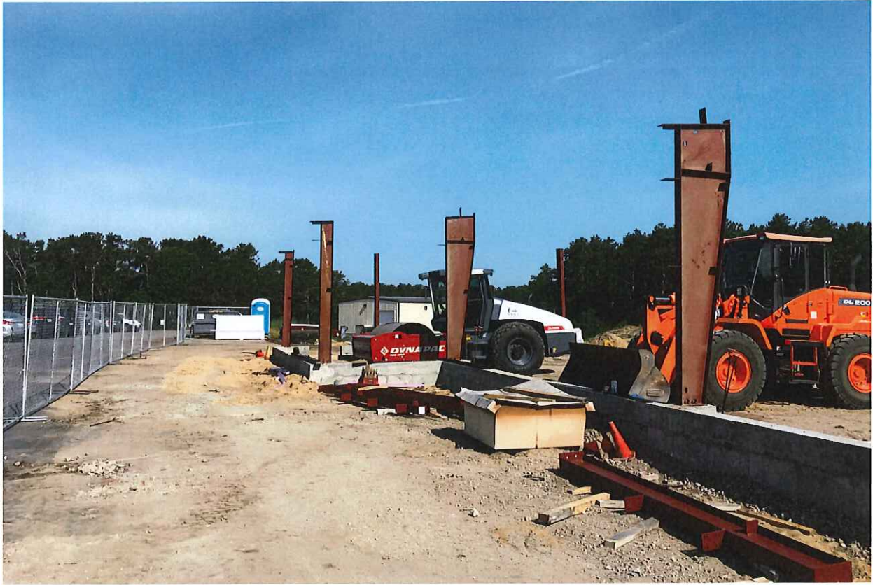
Steel supports for superstructure
