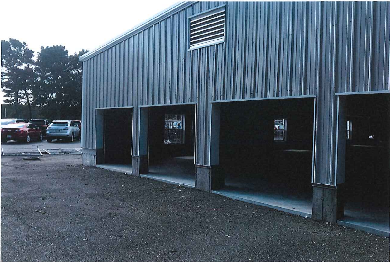
Front View of the new Cart Barn
