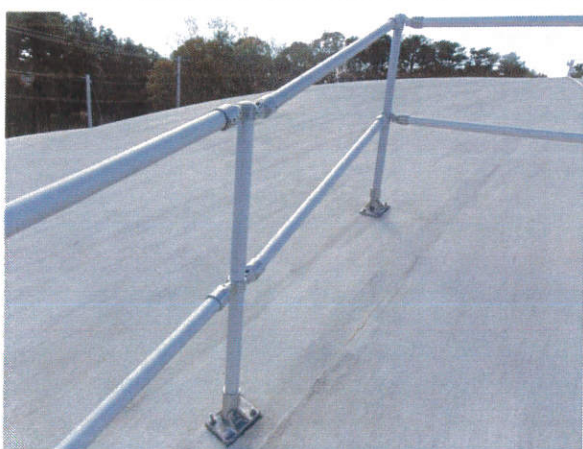
9) Roof safety railing
