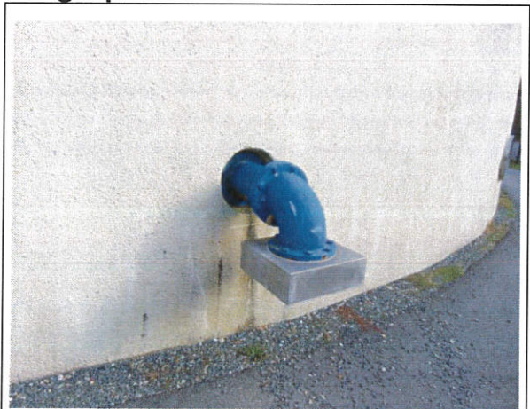
4) Overflow pipe tank termination
