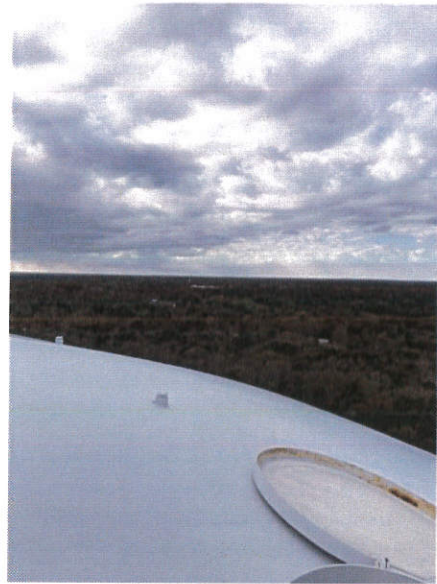
14) General roof view
