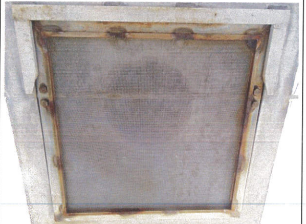
5) Fine mesh protective overflow screen
