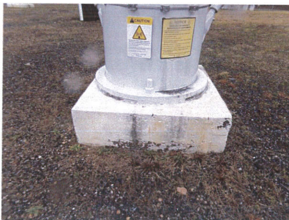
3) Typical view of leg base
