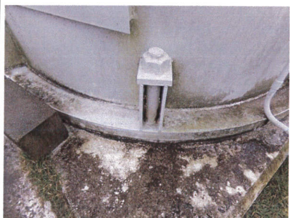
6) Close up of anchor bolt for riser pipe
