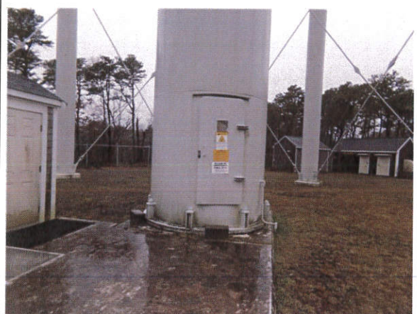
5) View of lower riser pipe
