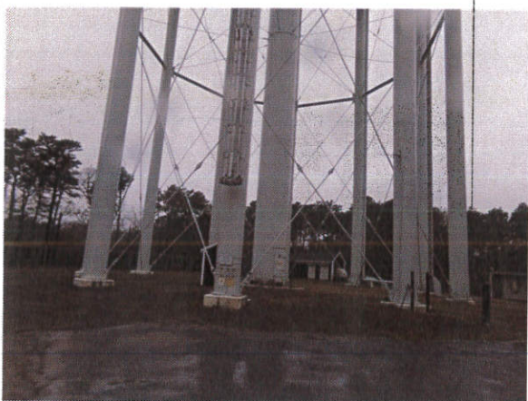
2) Lower portion of tank
