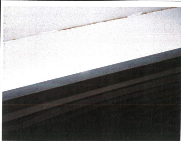
20) Close up of typical roof beam
