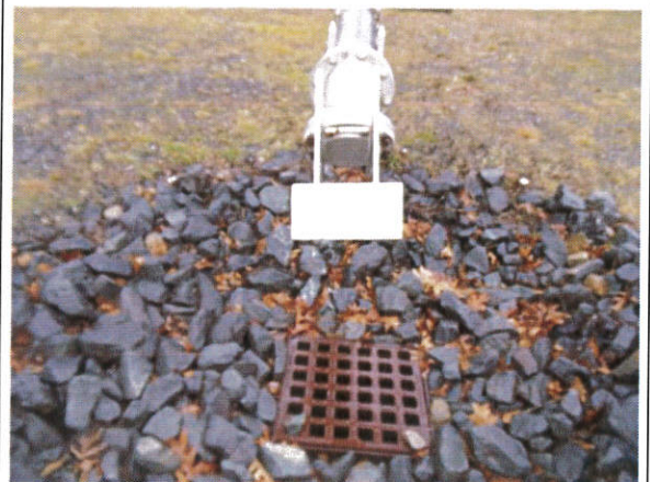
10) Overflow termination with grate for drain
