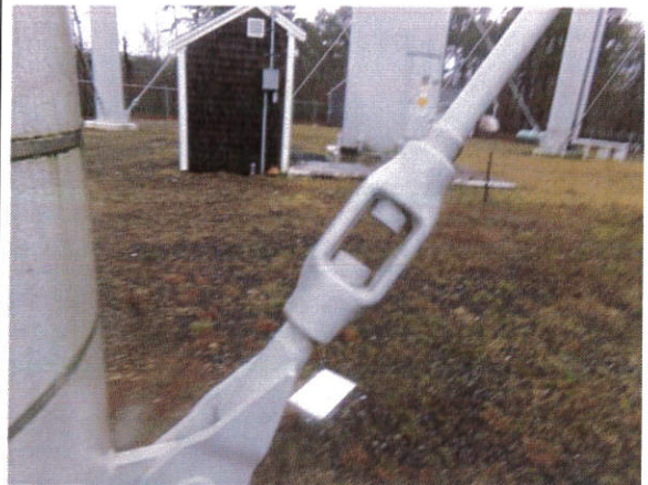
4) Typical turnbuckle connection
