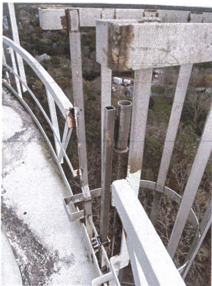
17) Balcony step off and top of leg ladder with safety cage
