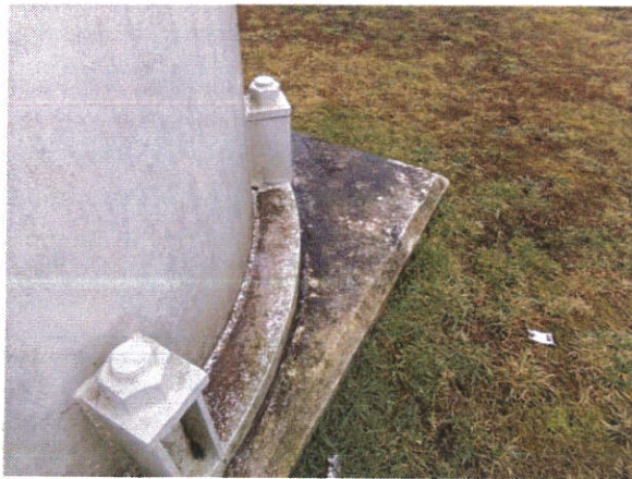
7) Riser pipe base with anchor bolts and foundation
