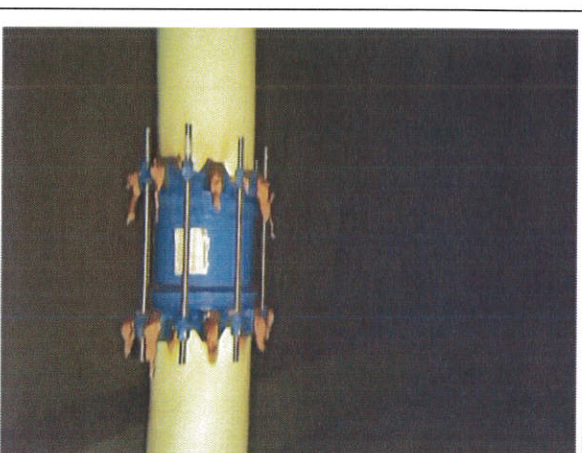
18) Repair clamp on inlet pipe 9:32
