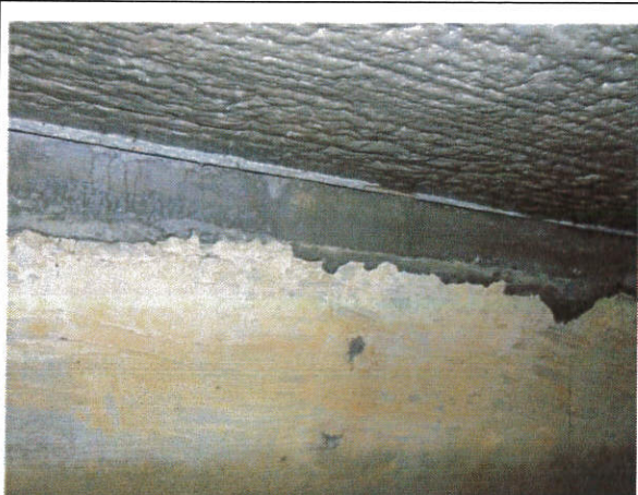
13) Closer view of interior roof to shell intersection
