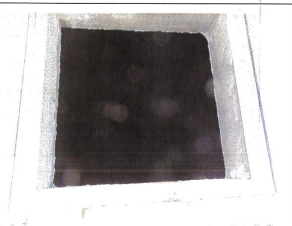
14) Roof manway opening
