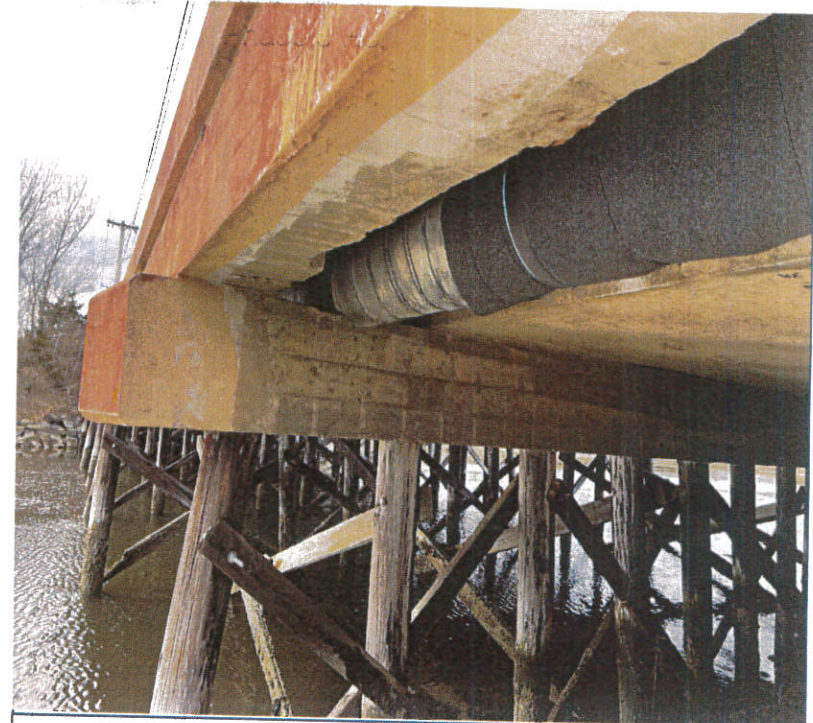
Phase 3 Herring River Bridge
