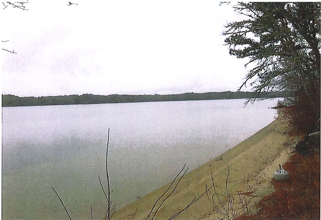
View to the east of Long Pond
