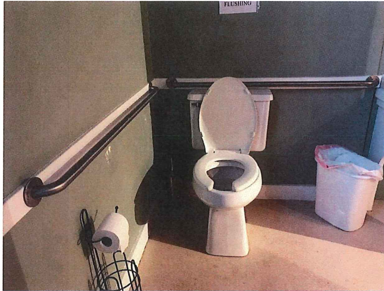
Figure 4 while the toilet room has accessible features, there required clearances for fixtures is inadequate
