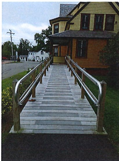
Photo 1 – Ramp with Non-Skid Surface
