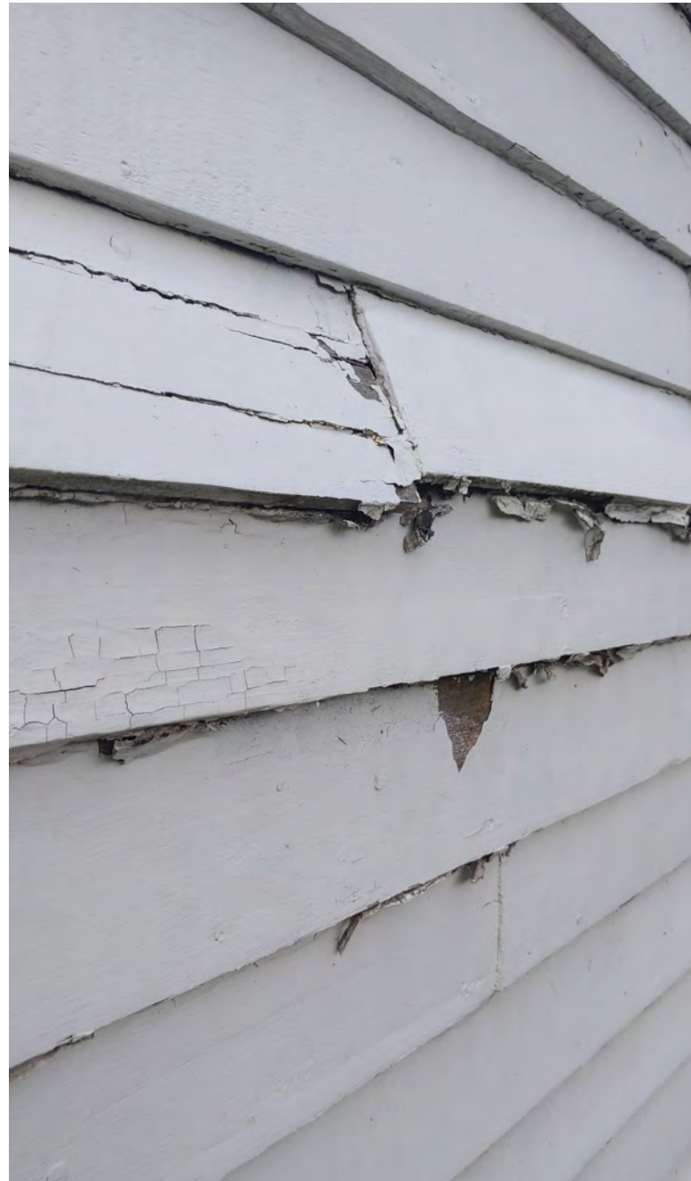
Peeling paint exposes wood cladding and trim to weather and rot.
