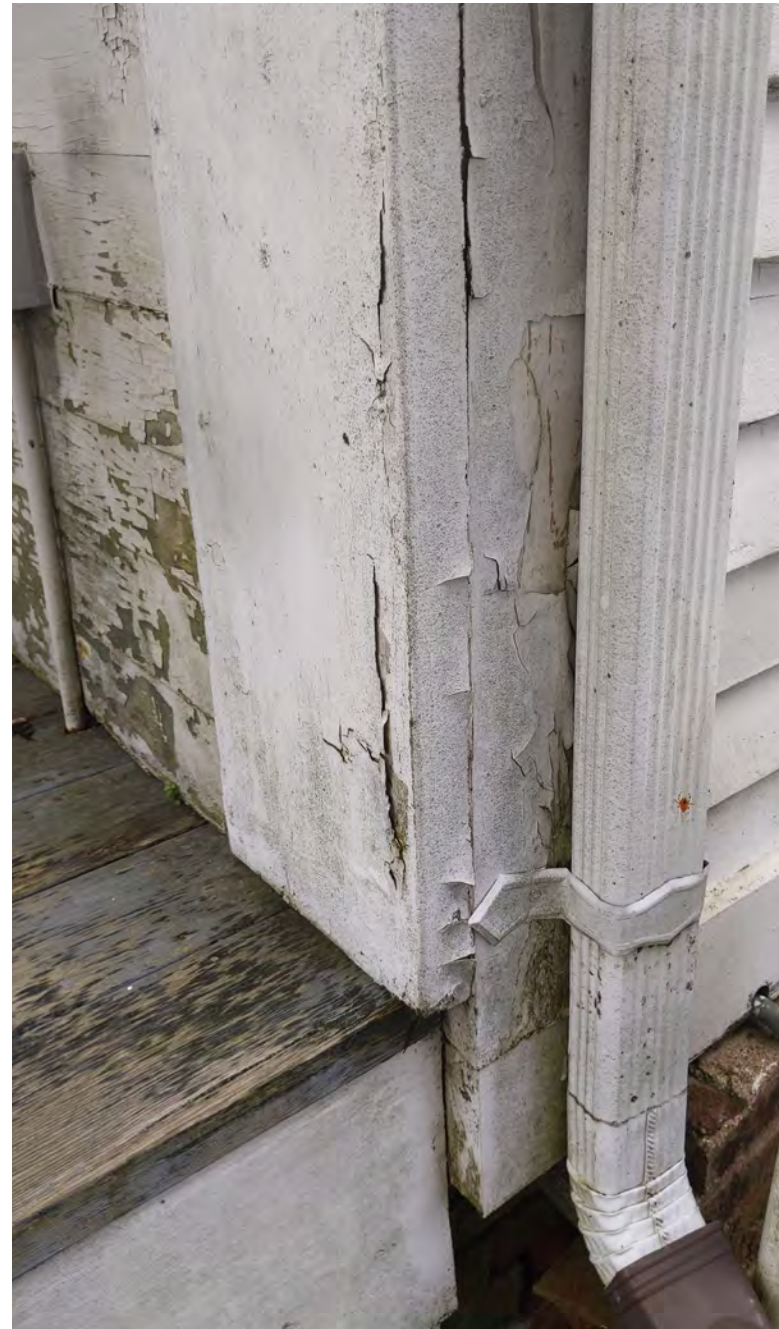
Peeling paint exposes wood cladding and trim to weather and rot.
