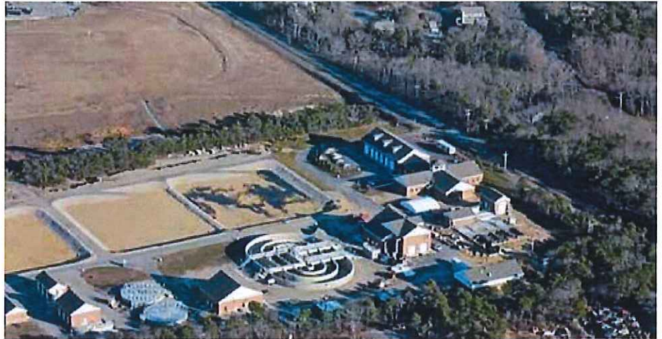
Chatham Wastewater Treatment Plant (1.3 million gallon per day average flow capacity with open infiltration recharge basins)
