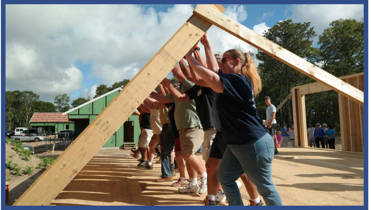
Habitat for Humanity Wall Raising, Summer 2016, Oak Street, Harwich
