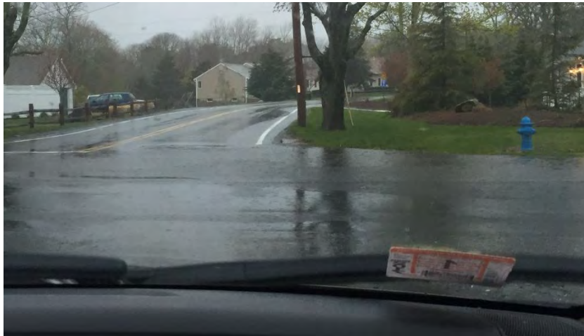
Figure 13 - Looking west, showing ponding during heavy rain event
