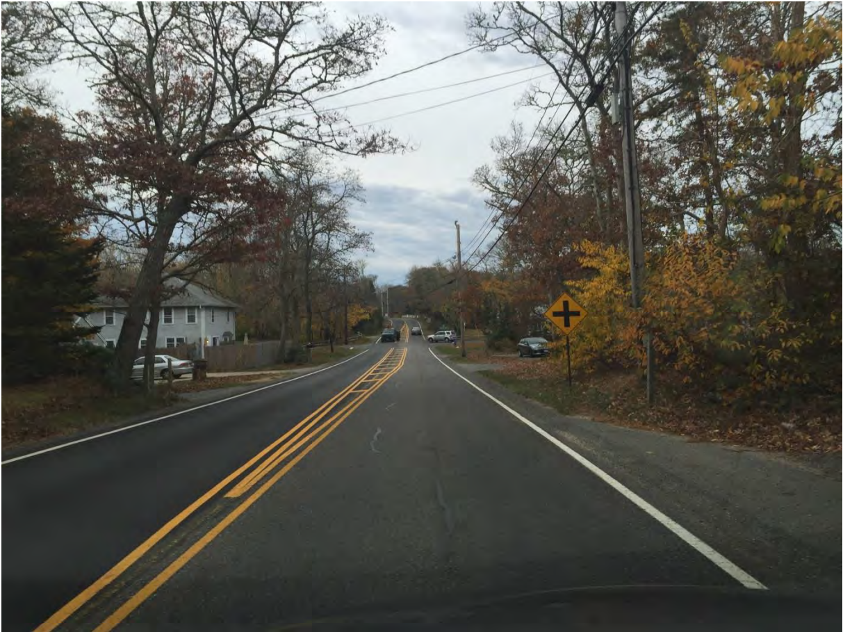
Figure 4 - View looking south, showing newly installed painted median
