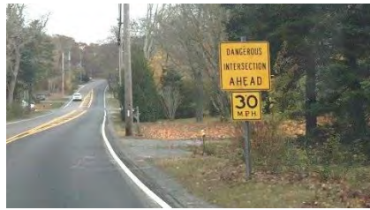
Figure 12 – Looking north on Route 39, showing current signage
