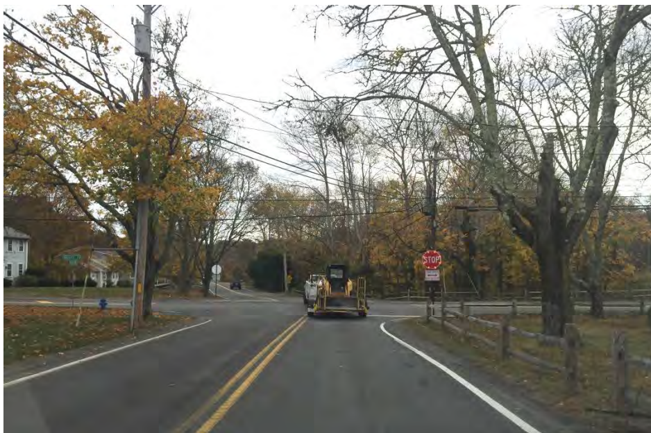
Figure 11 – Looking east on Pleasant Bay Road, showing LED stop sign
