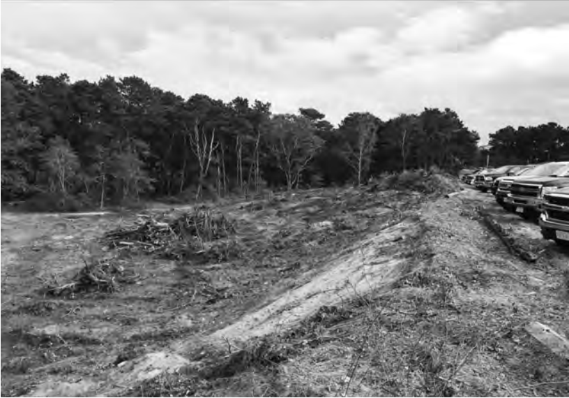
Site preparation for the new “Cart Barn”
