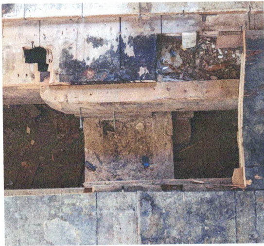
FRONT TWO CHIMNEYS, SHOWING STEEP ANGLE OF COBBLING AND POOR SUPPORTS
