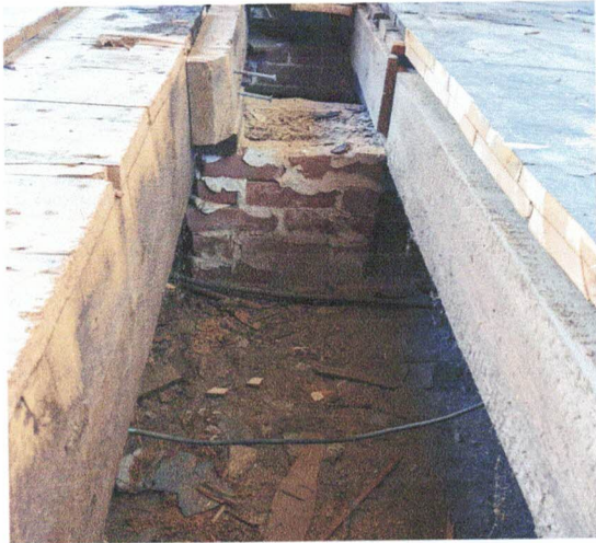
ORIGINAL REAR CHIMNEY FOOTING UNDER KITCHEN FLOOR
