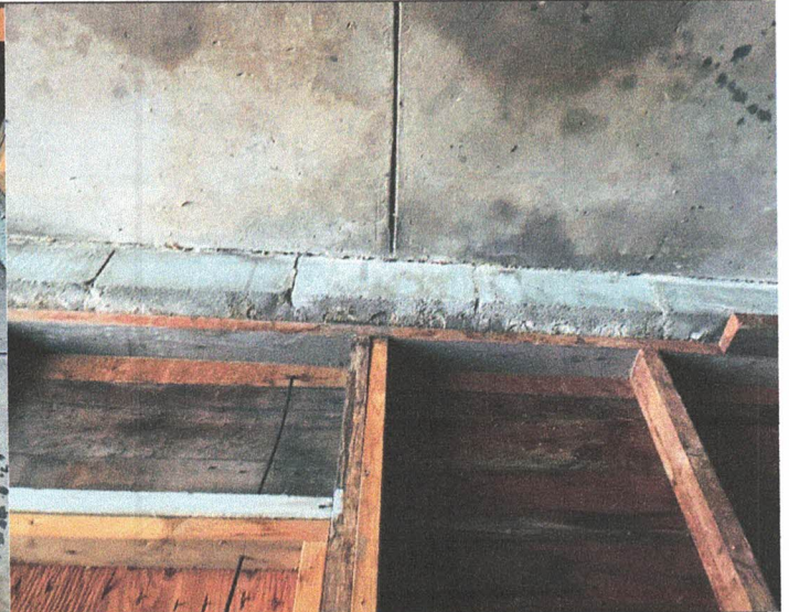
P10: Concrete block with grout infill as garage curb.
