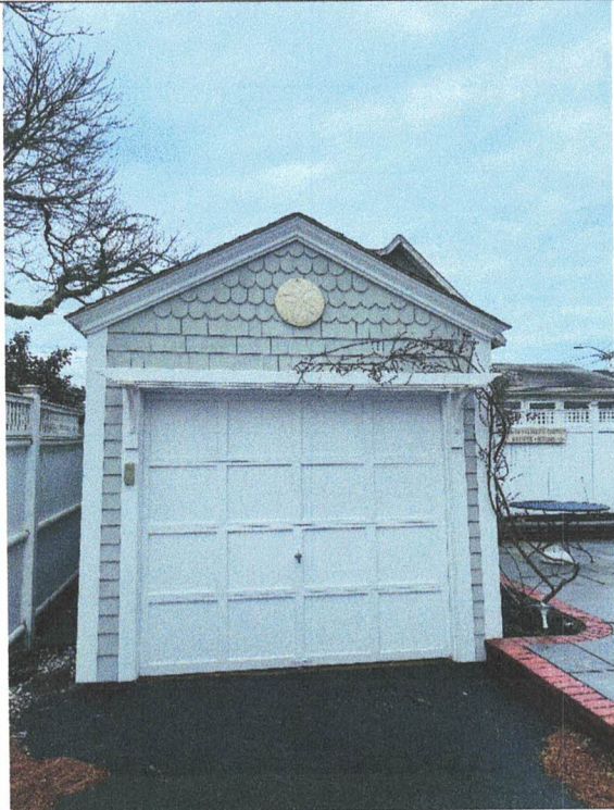
P1: Gable pitch roof with scallop shingles and crown fascia
