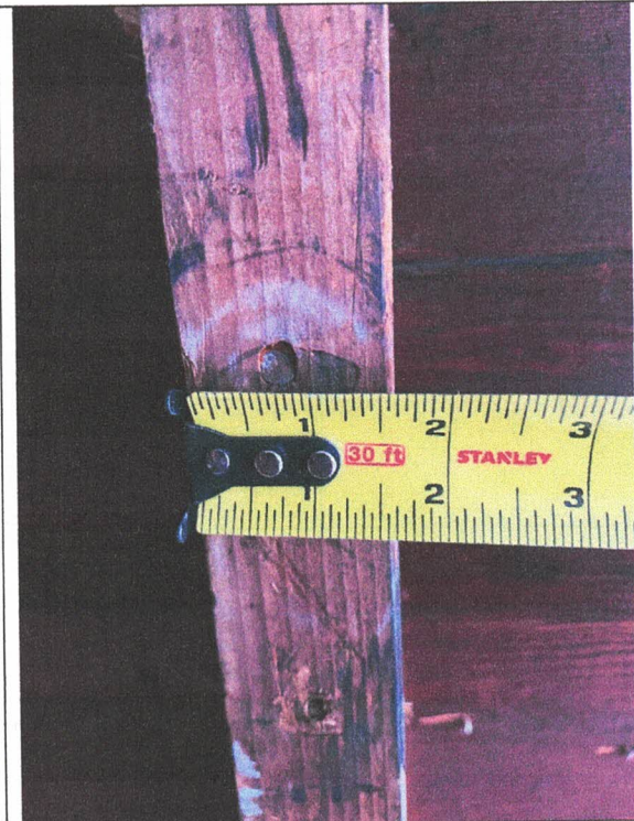
P5: 2x Stud thickness(1-1/2")
