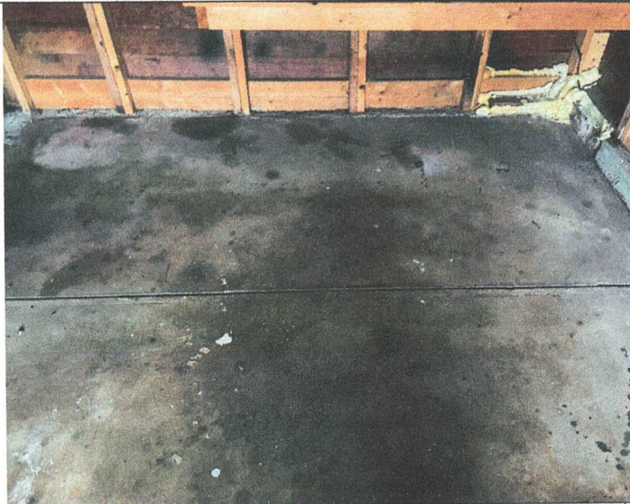
P9: Concrete garage slab
