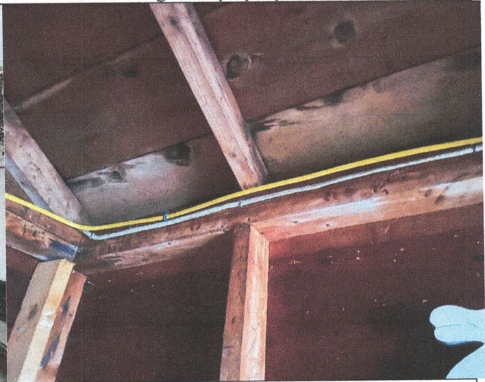
P4: Double top plate & 2X rafters/studs @24"OC
