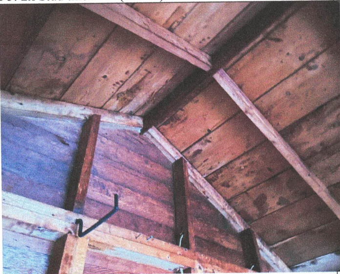
P5: 2x Stud thickness(1-1/2")
