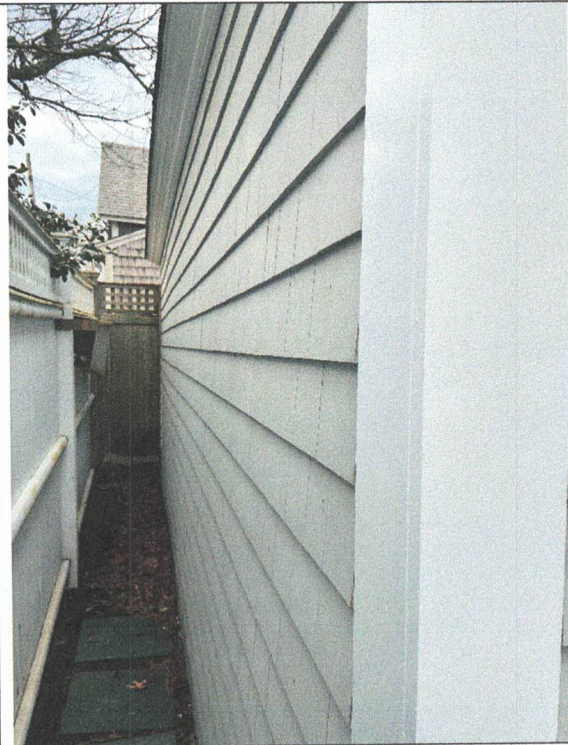
P2: North wall along fence/property line
