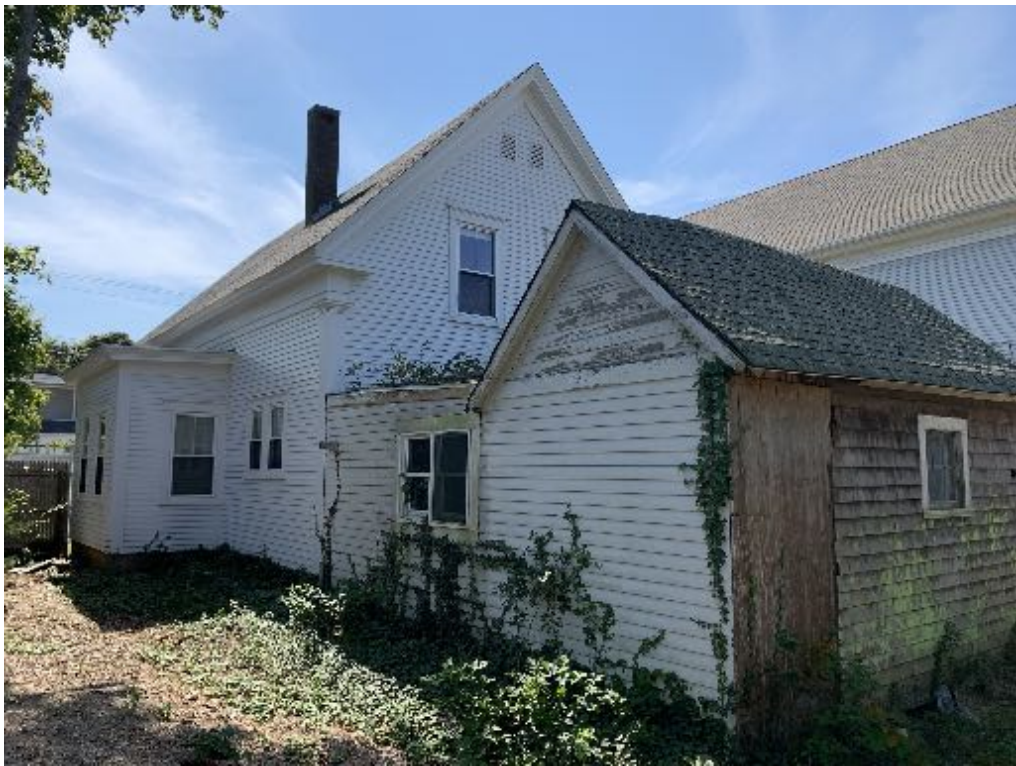
North - East View of the House
