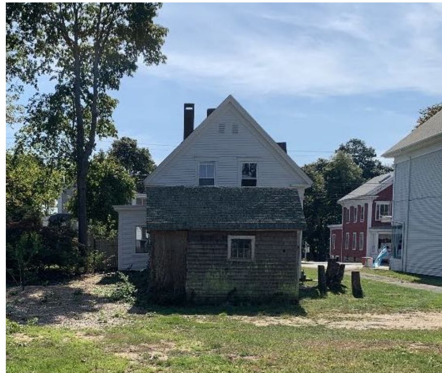
North View of the House
