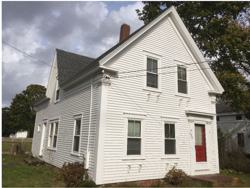
South - West View of the House
