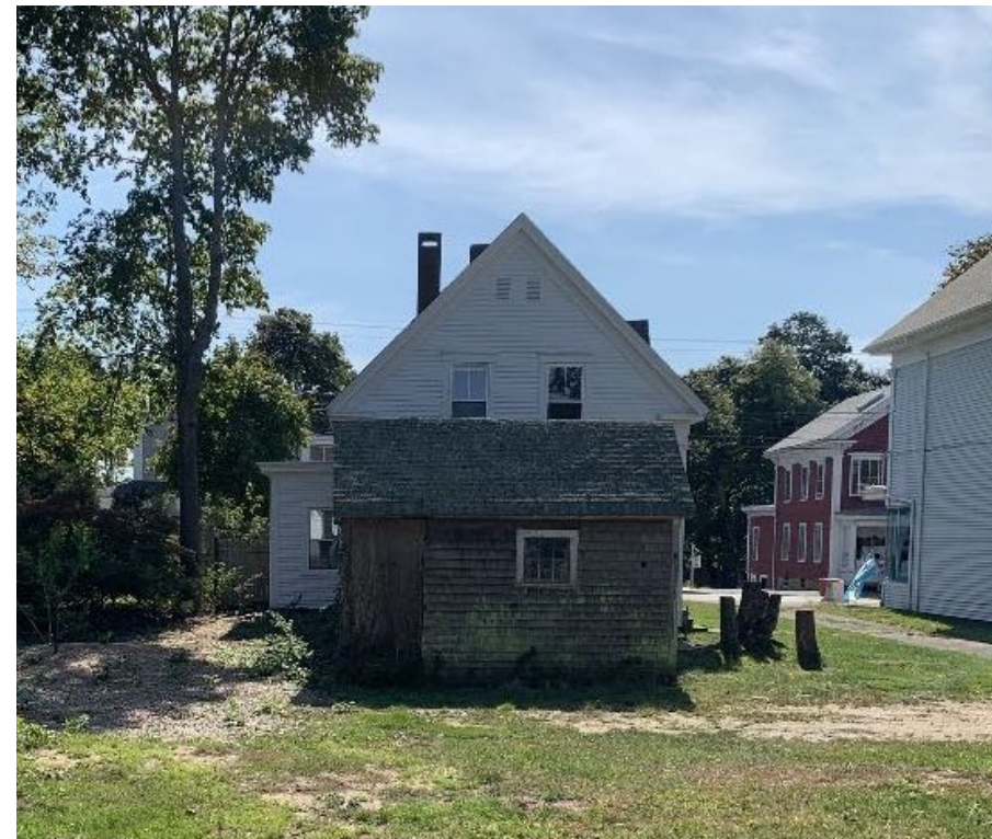
North View of the House
