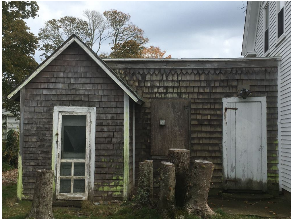
South View of the Shed and Connector
