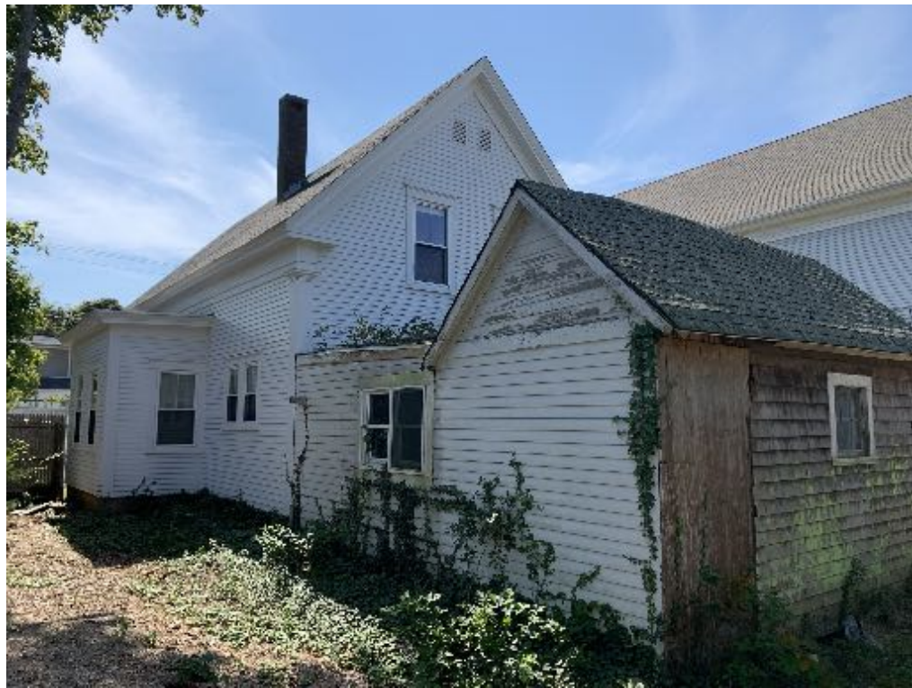
North - East View of the House
