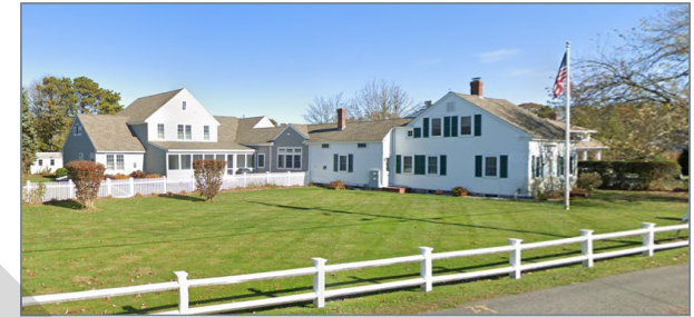
Additions to this historic building have pitched roof forms and lower ridge heights to make them secondary to the historic building. Larger forms are placed to the rear where they have less impact on the original building scale. Image: Google maps.
