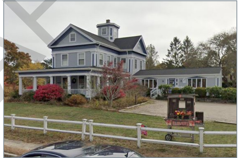
A one-story shop was added to this circa 1840 building without altering its original building form and many architectural details. Image: Google maps.
