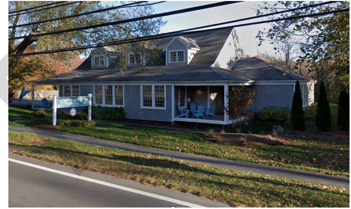
This design includes multiple building masses, changes in roof form, and low eave heights to respect traditional building forms nearby. Image: Google maps.
