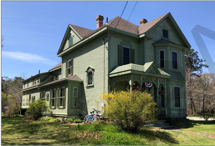
The Captain Bearse house maintains its circa 1890 Queen Anne style porch, bay windows, and cornices, as well as its series of rear additions.
