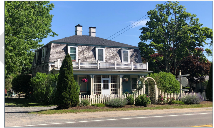
The glass enclosure added to the entry of this historic home can be removed without destroying the original porch or facade details.
