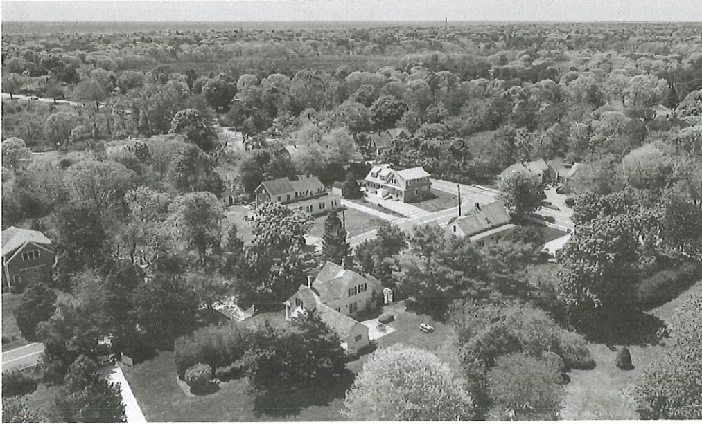
Birdseye View (North Elevation)
