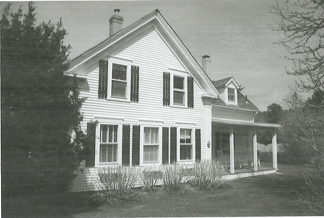
South Elevation (8 Gorham Rd / Street View)
