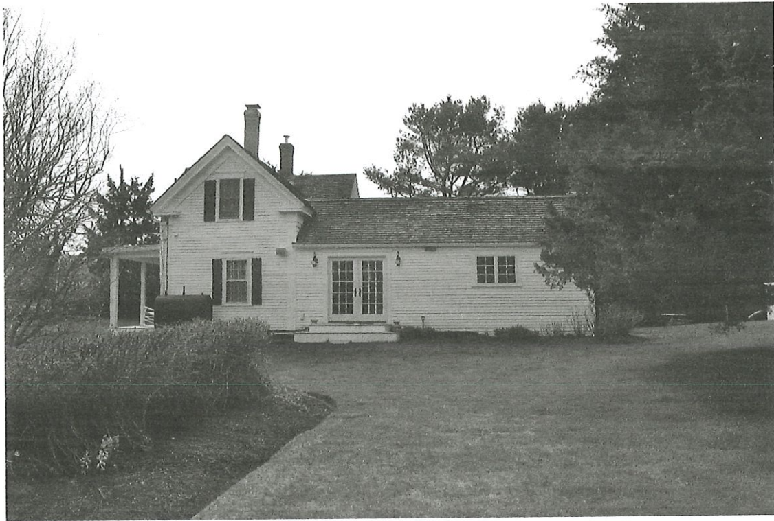
East Elevation (Right Side)
