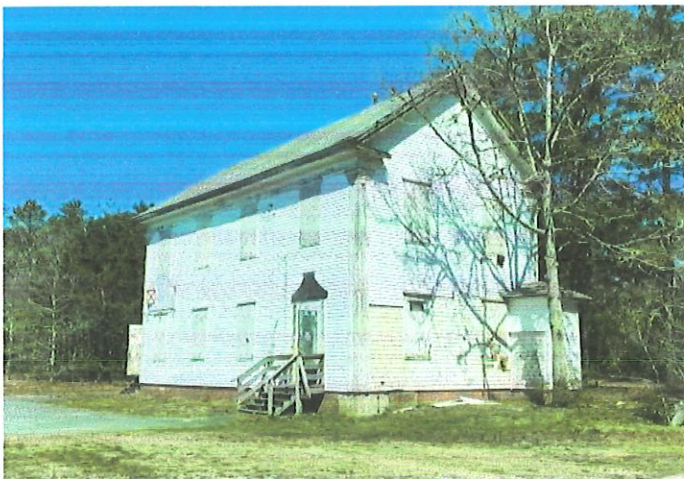
South and East Facade
