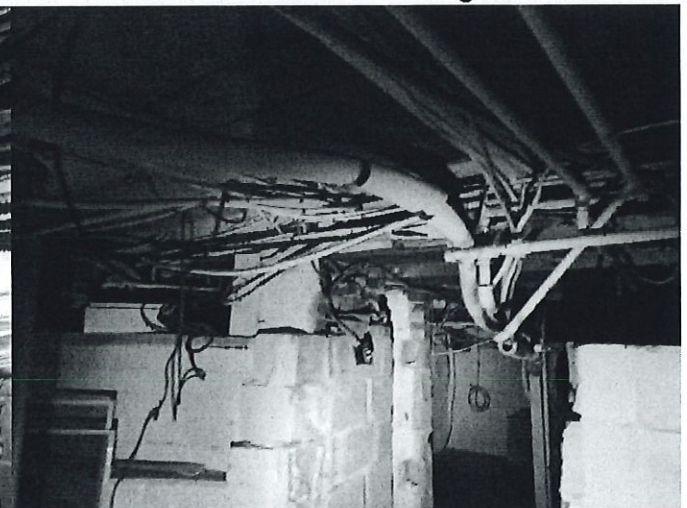
Photo 6: First floor framing and floorboards
