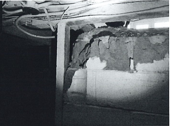
Photo 4: CMU wall with framing above
