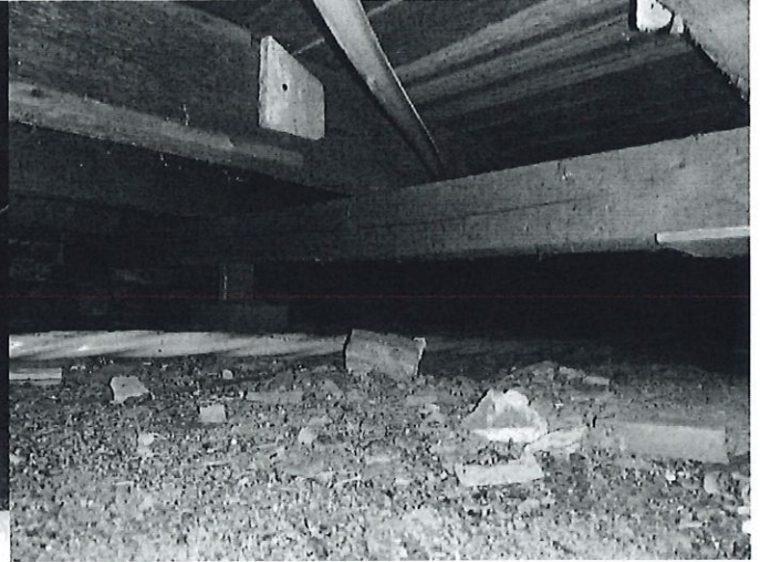
Photo 2: Exterior wall and support at crawlspace
