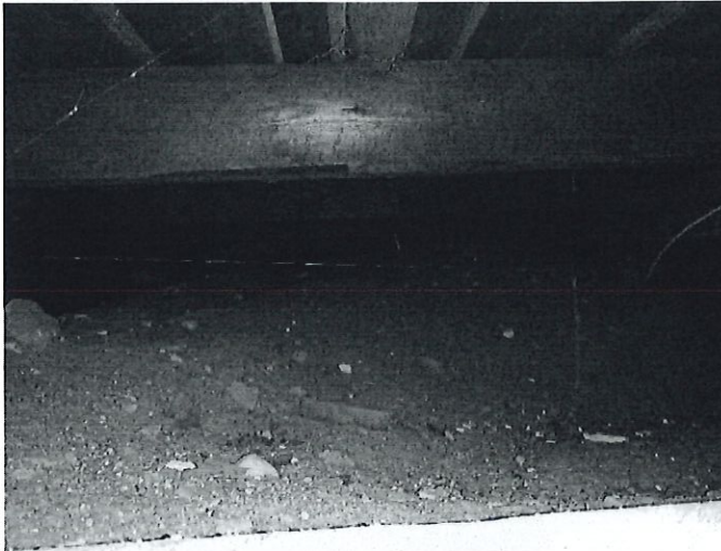
Photo 1: Framing at crawlspace
