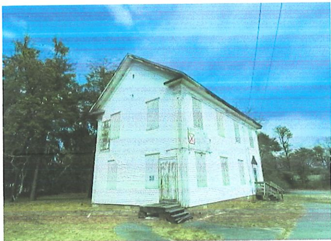
South and West Facade
