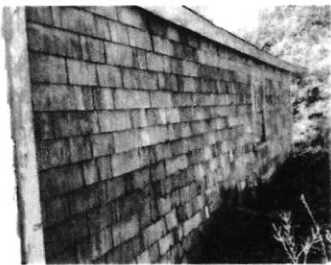
P5 EXISTING PHOTO: REAR FACADE 1/4" = 1'-0"
